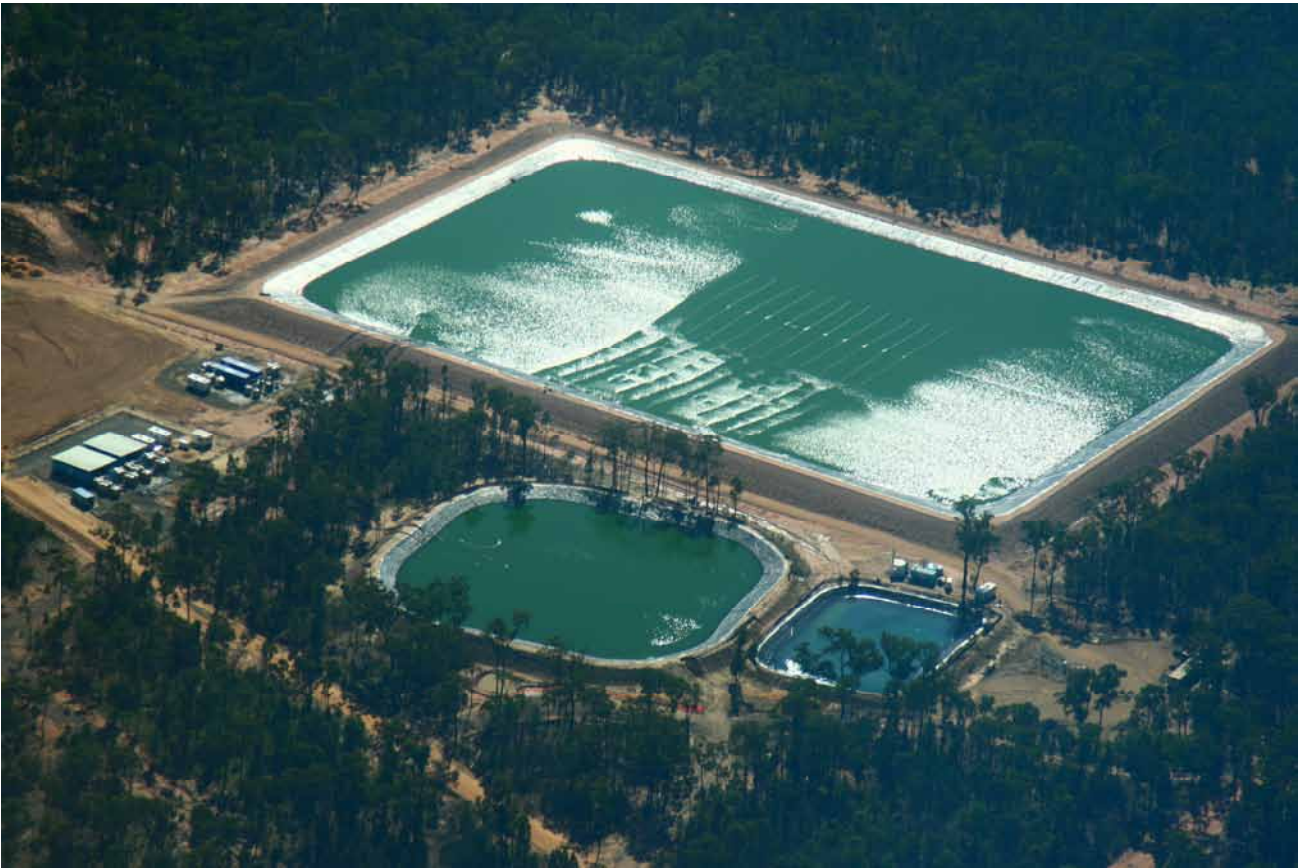
Bibblewindi Treatment Plant. Photo: T.Pickard.
